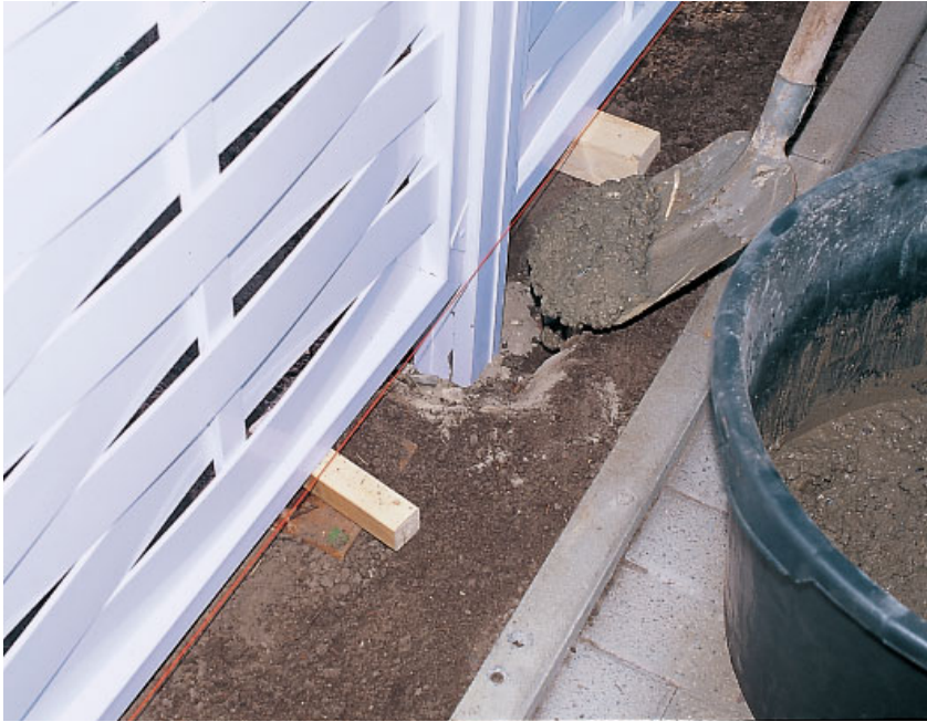
Palen direct in de aarde inbetonneren...
